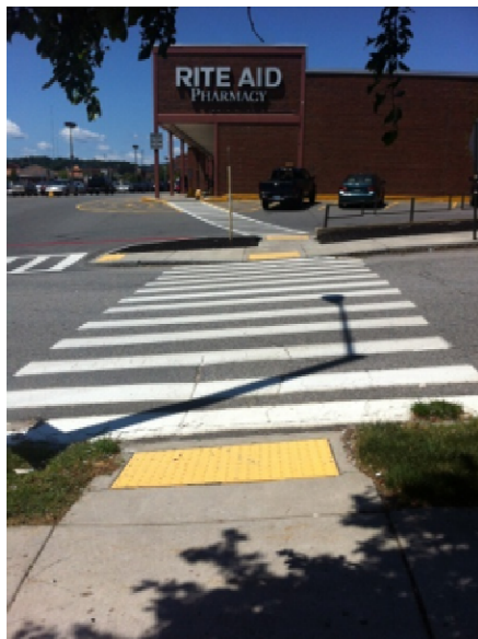
Photo: An example of an ADA ramp with detectable warning tactile surface.
